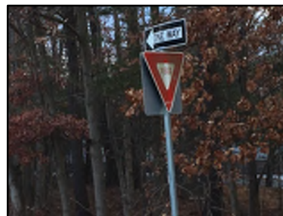
Image 6: Murky YIELD sign along Frontage Road.
